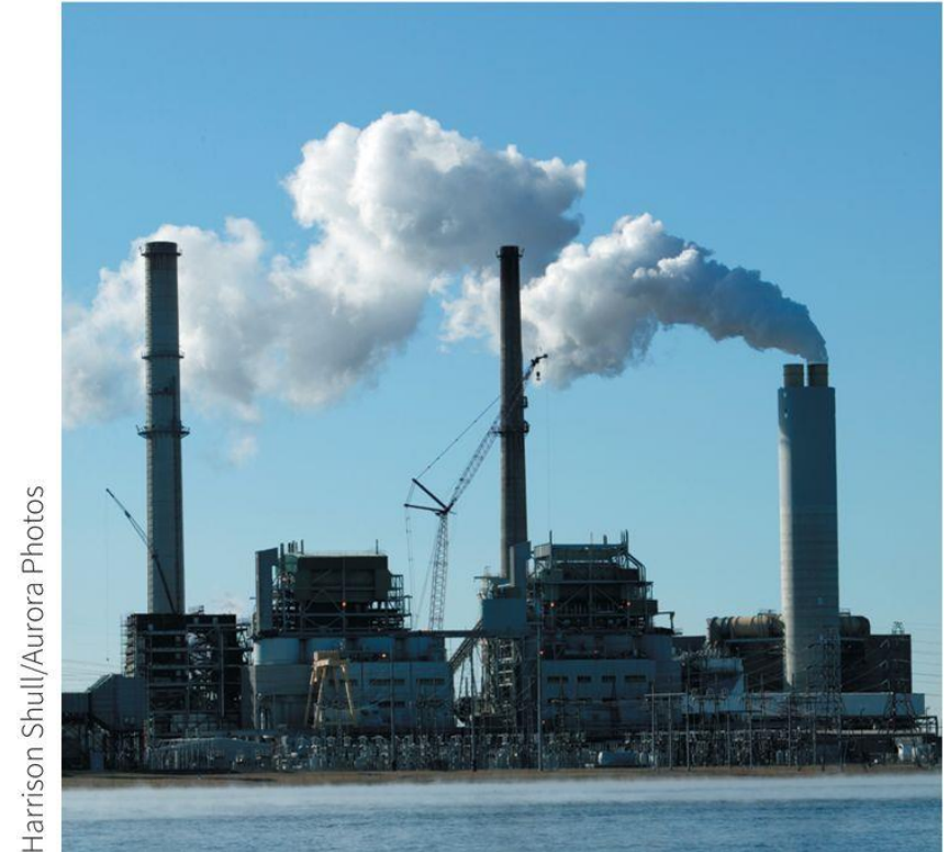
Emissions controlled with scrubbers-only steam expelled (North Carolina)
